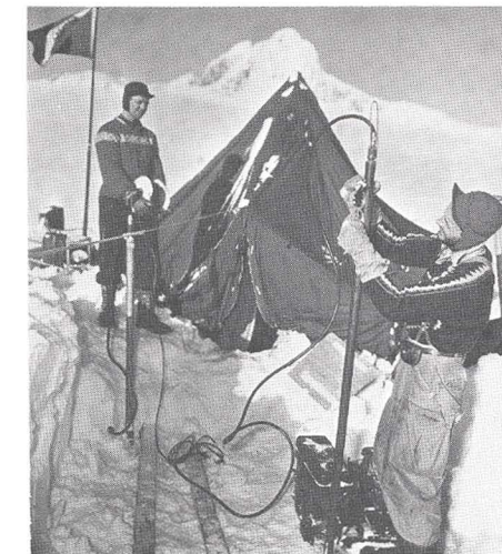
Electro-thermic glacier drilling on the Juneau Icefield.
